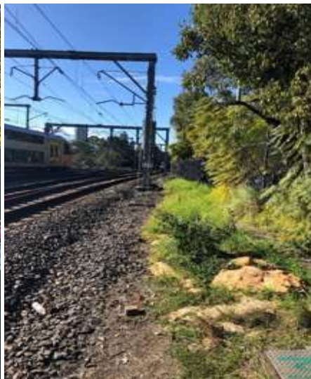
City side of Hut Down Cess
