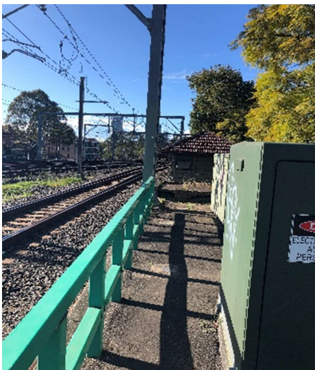
Inside gate W00 25.073 Down Cess
