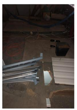
An ARTC worker was showing a contractor where to set up cabling in the roof space. Whilst walking on the designated mezzanine walkway in the roof space the worker has stepped through the walkway and the ceiling. Fortunately, only one of the worker's legs has penetrated through the walkway and ceiling. The potential fall risk was approximately 5 metres. The worker was able to remove himself and was not injured but there was potential for significant or fatal injuries.
