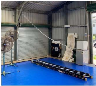
Incident scene post incident. The base of ladder has slipped and kicked out beneath worker.
