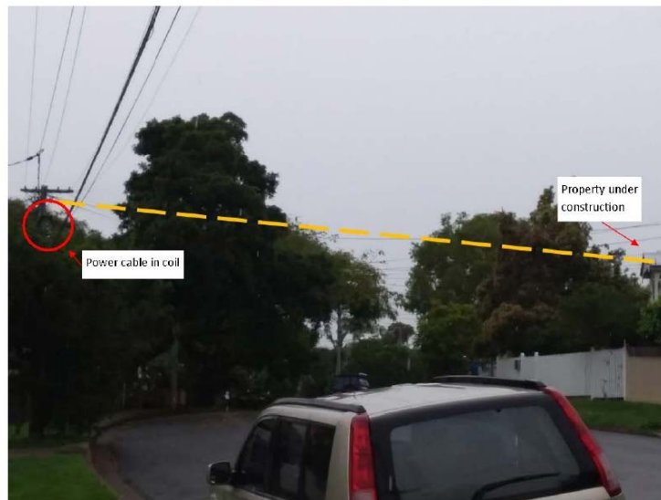
Figure 1 and 2. Power cable removed from dwelling and coiled onto adjacent Power Pole
