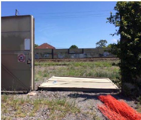
Right hand sound wall gate
