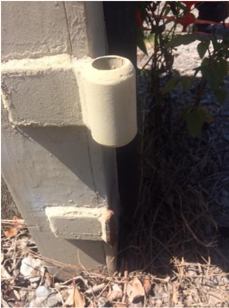
Lower hinge pin support bracket
