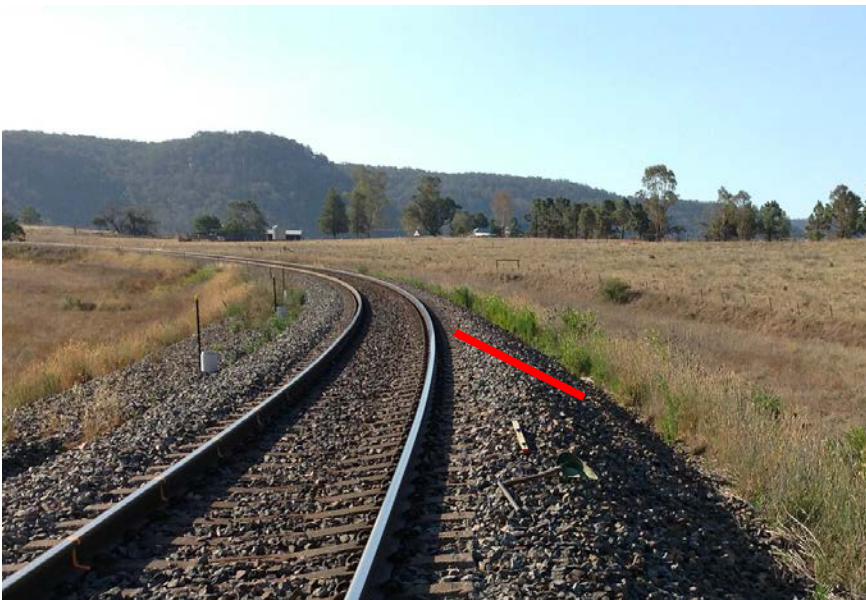
Image 3: Red line indicates cross level board being stored on ballast shoulder. The left hand edge was struck by the train.
